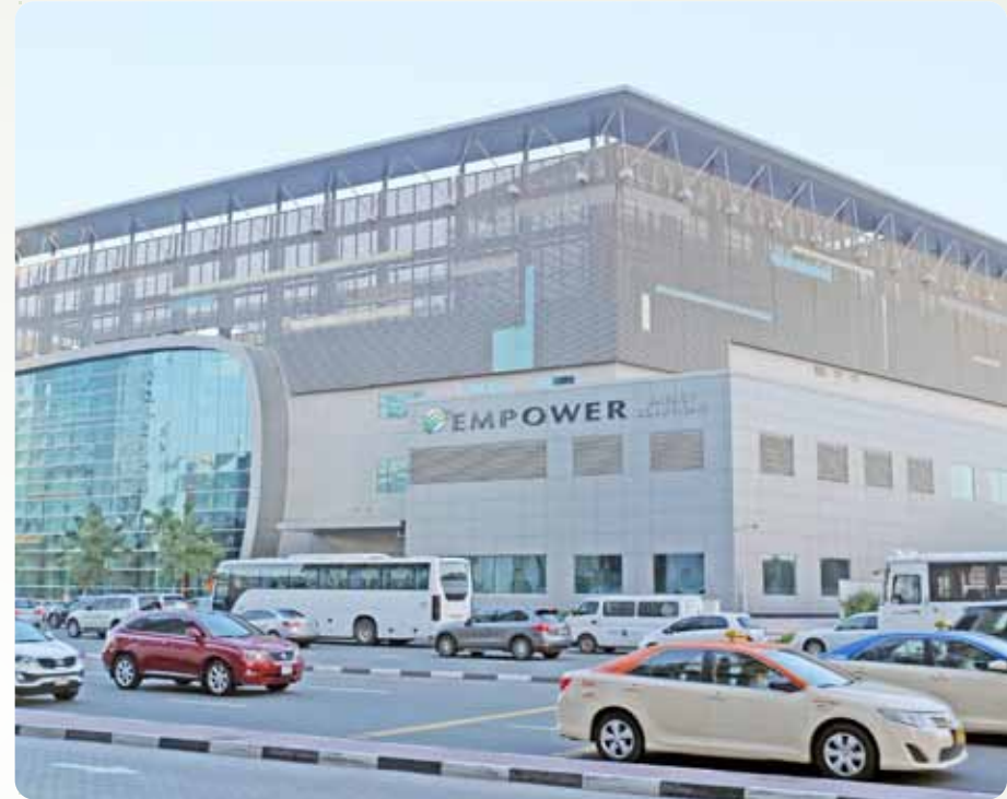
Empower's district cooling station, Dubai
