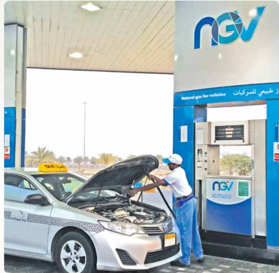
CNG pumps at an ADNOC station
