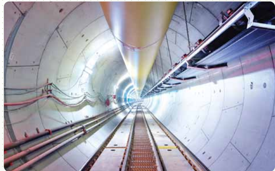
A sewer tunnel under construction in Abu Dhabi
