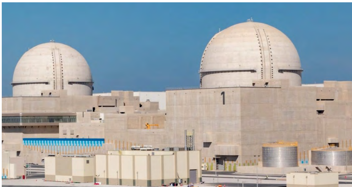
Barakah Nuclear Energy Plant
