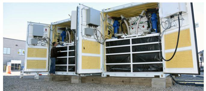
Figure 5. Flow battery at Idaho National Laboratory's Microgrid test bed. Source: U.S. Department of Energy
